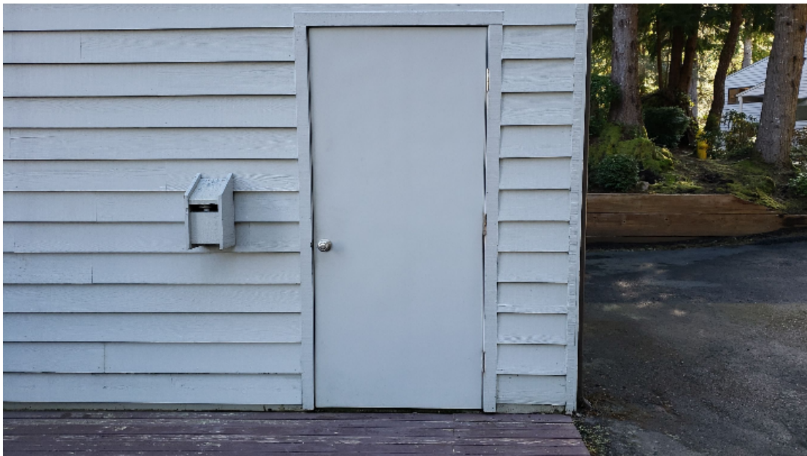
Building Exterior - Doors, Garage Side & Courtyard
