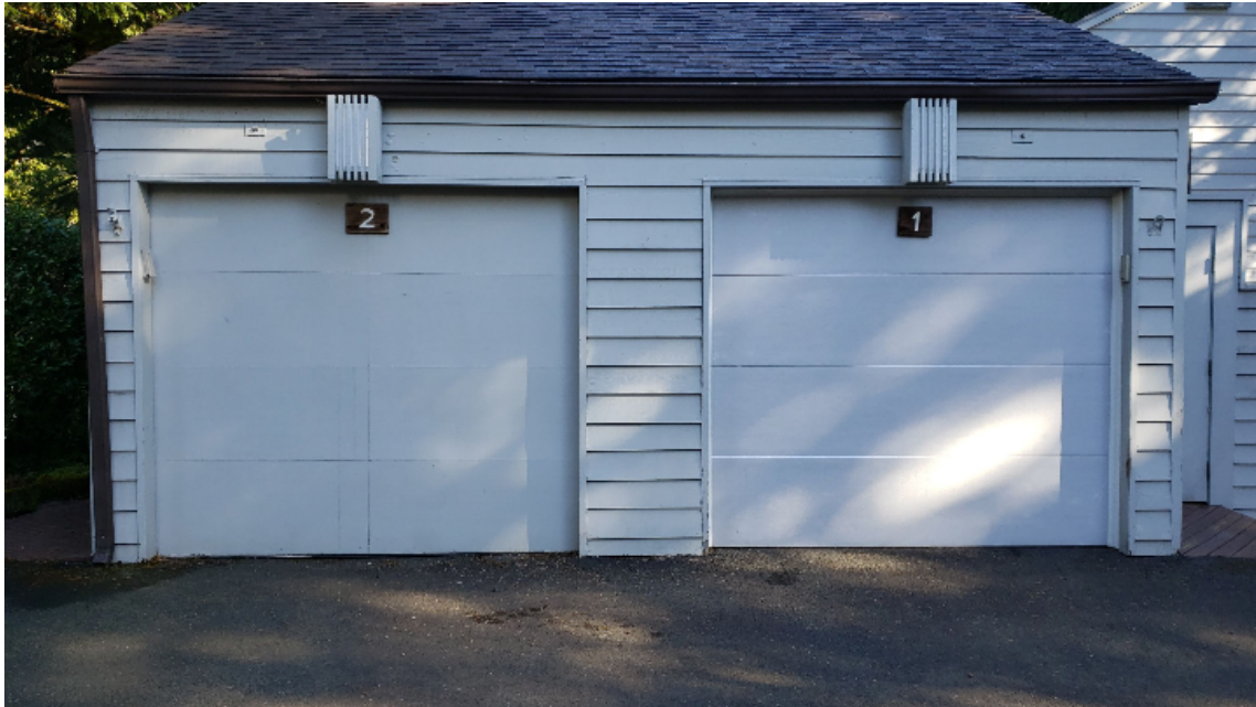
Building Exterior - Garage Doors
