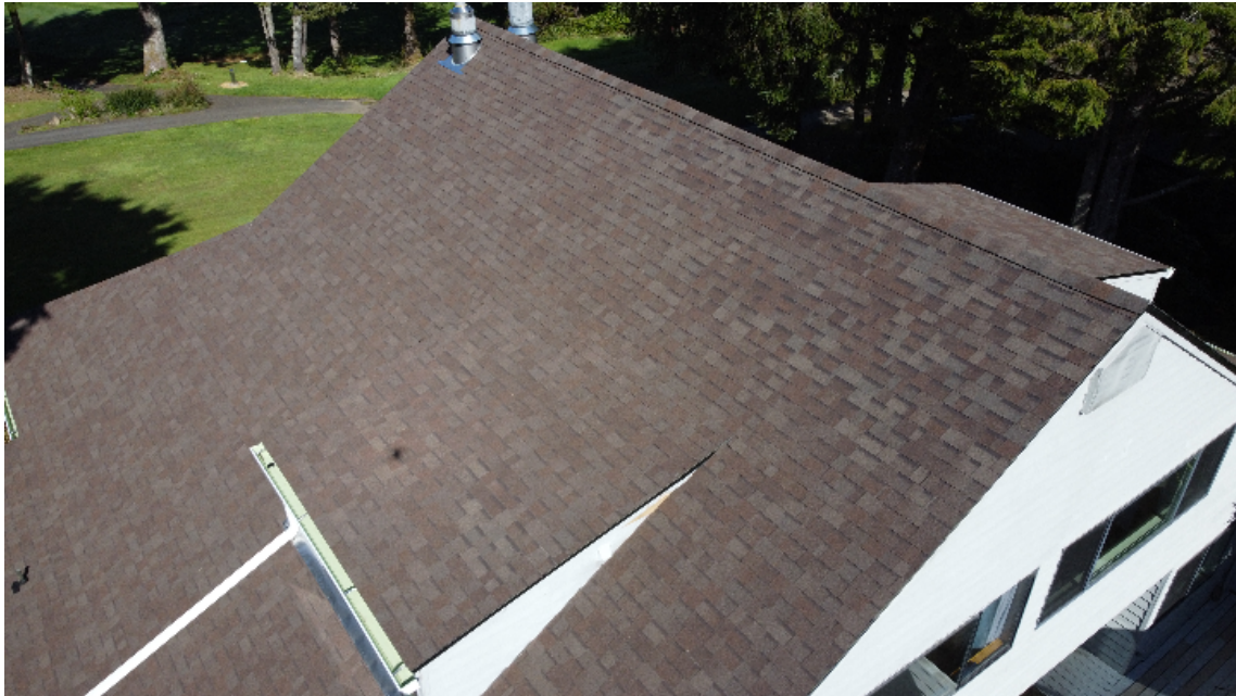
Building Exterior - Roof, Asphalt Shingle, Units 11 & 12
