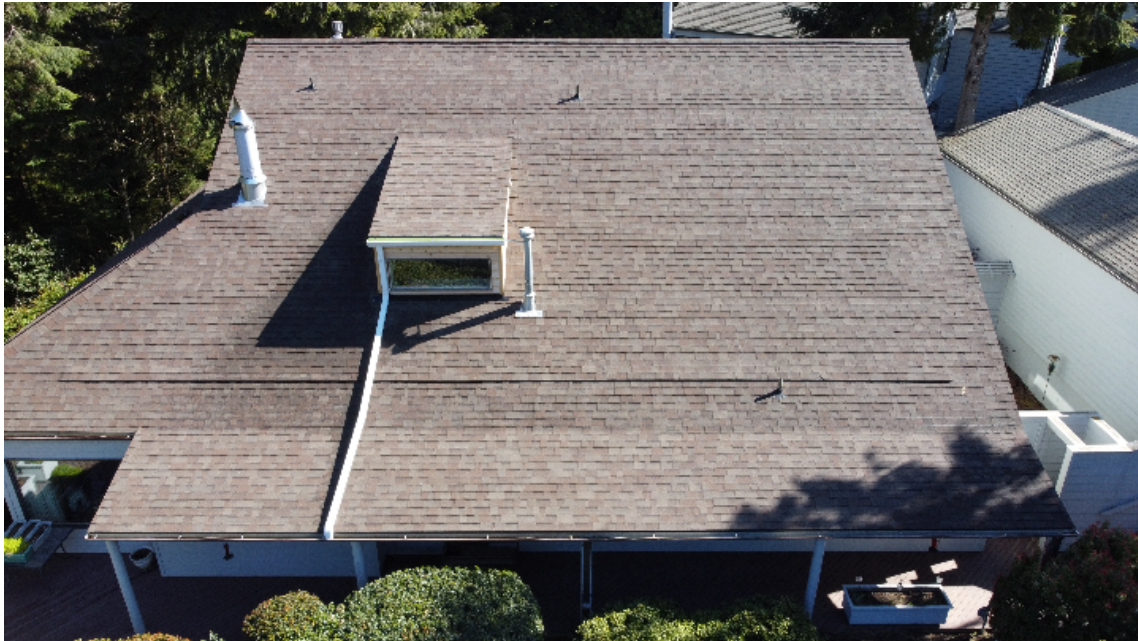
Building Exterior - Roof, Asphalt Shingle, Units 7 & 8
