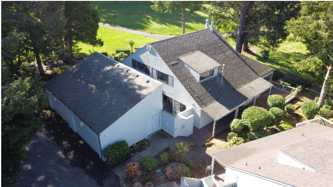
Building Exterior - Roof, Units 15 & 16 Garage
