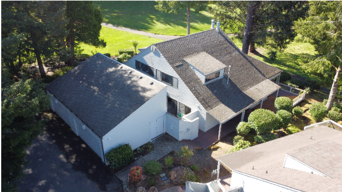
Building Exterior - Roof, Asphalt Shingle, Units 15 & 16
