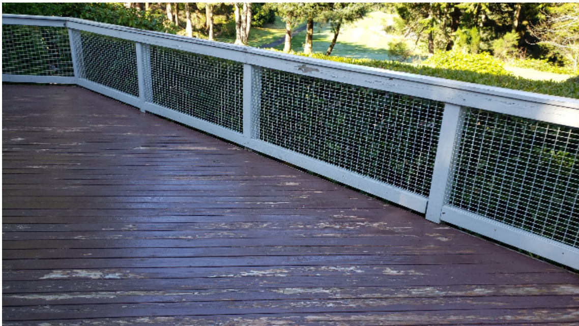
Building Exterior - Deck, Guardrail, 25% Replace
