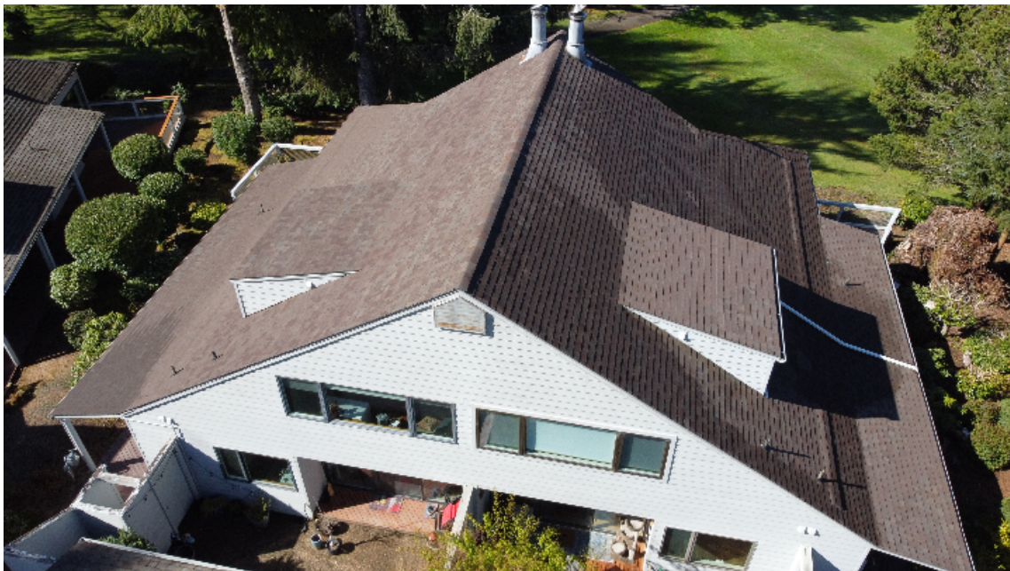
Building Exterior - Roof, Asphalt Shingle, Units 13 & 14
