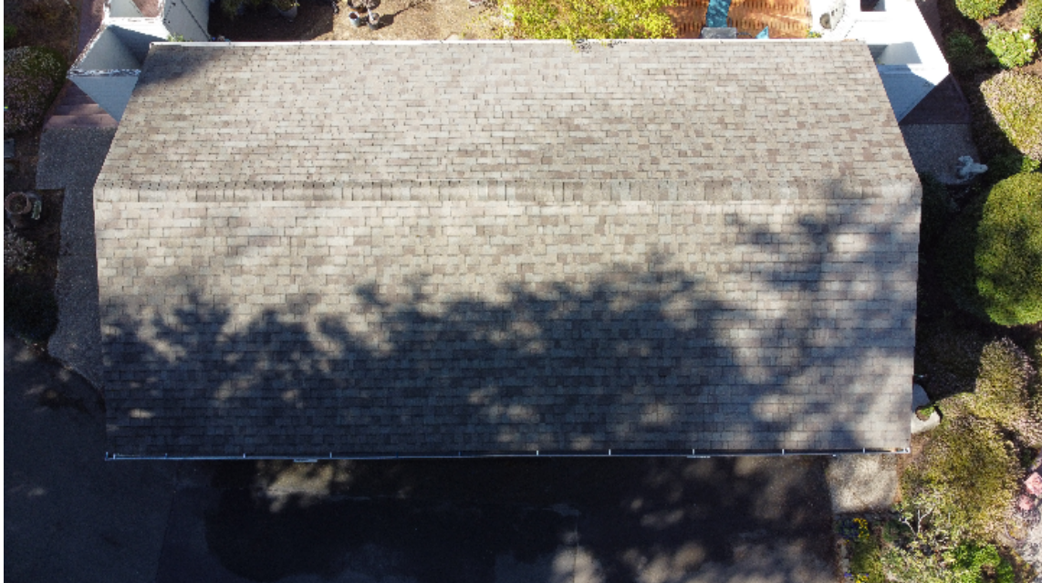
Building Exterior - Roof, Units 13 & 14 Garage
