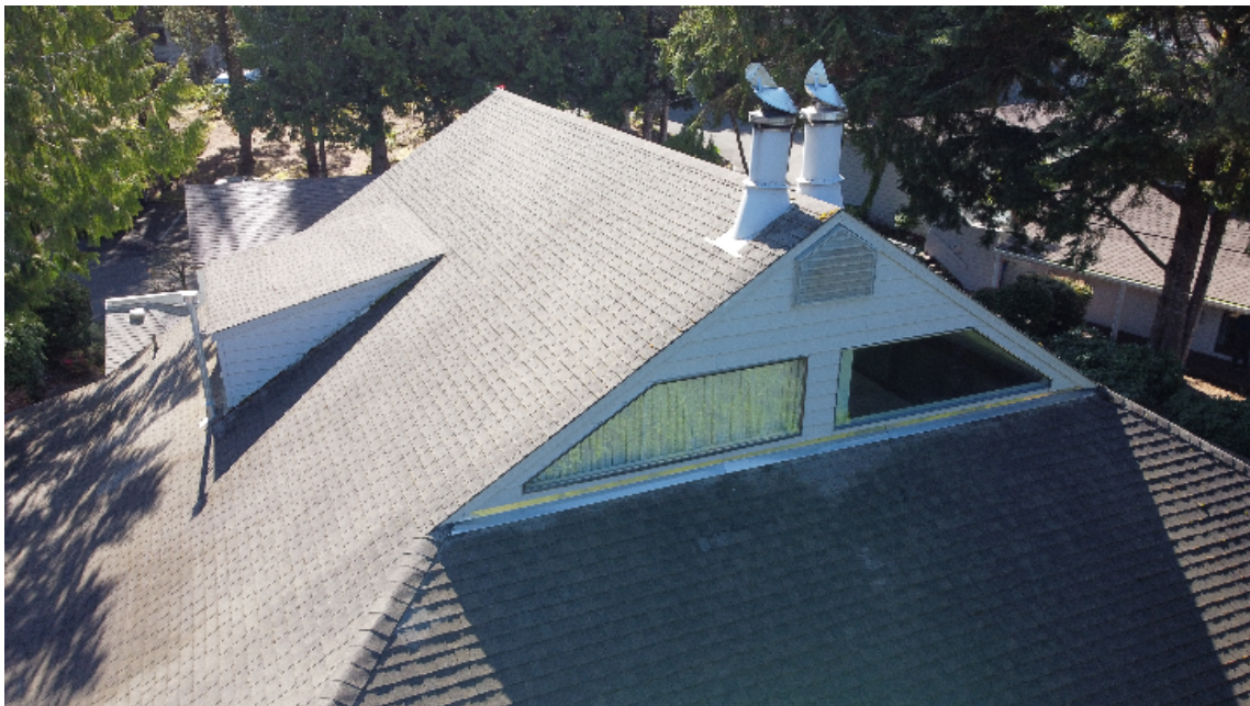
Building Exterior - Roof, Asphalt Shingle, Units 9 & 10
