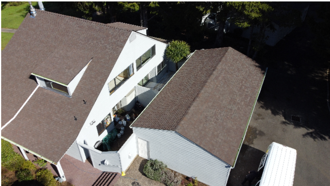
Building Exterior - Roof, Units 11 & 12 Garage
