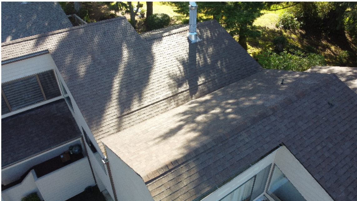
Building Exterior - Roof, Asphalt Shingle, Units 17 & 18
