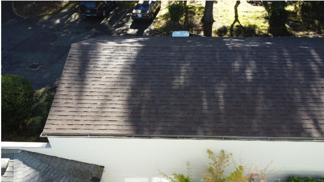
Building Exterior - Roof, Units 9 & 10 Garage
